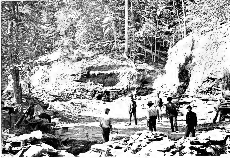
A GENERAL VIEW. DUCK RIVER PHOSPHATE COMPANY.
